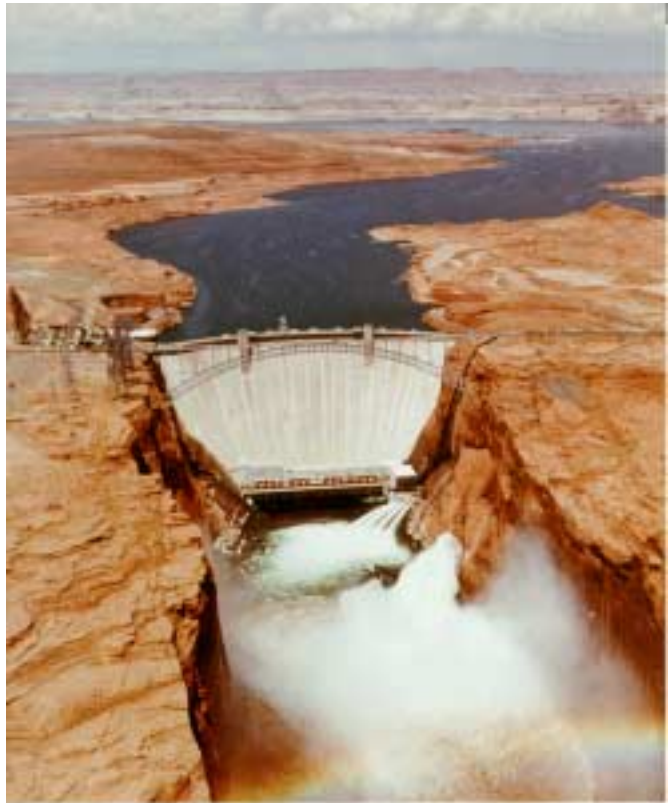
Glen Canyon Dam
