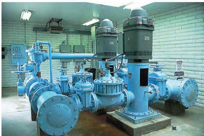
Where infiltration basins are not feasible, pumps can be used to inject water directly into the receiving aquifer. In some cases, the same pumps can also be used to recover the storage.
