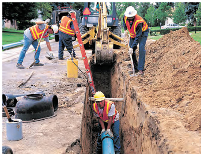
In some water systems, finding and repairing leaks may be the most desirable conservation alternative. Water savings from such measures are relatively easy to quantify.
