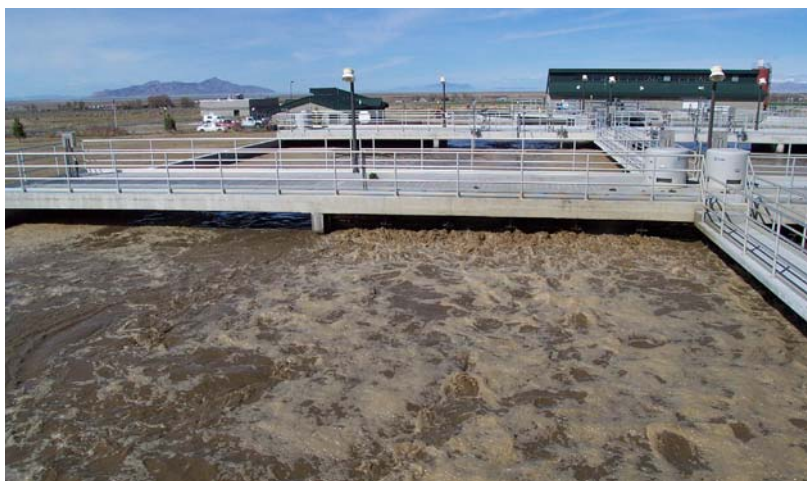
Tooele's wastewater treatment facility uses an oxidation ditch as part of its treatment process. (Photo courtesy of Tooele Wastewater Treatment Plant.)
