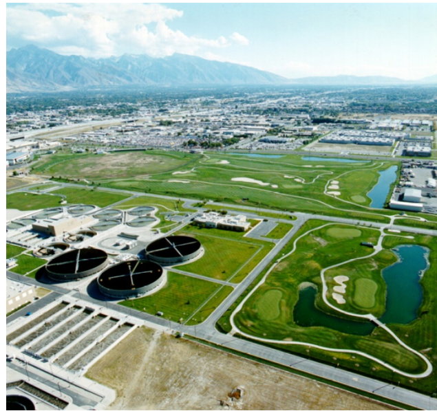
The Central Valley Water Reclamation facility reuses the treated effluent to irrigate an adjacent golf course and is a centralized reuse system.
