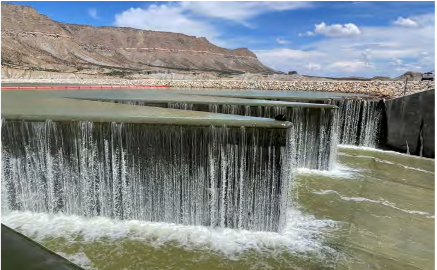
Millsite Reservoir spillway, a board-funded project completed in 2023.
