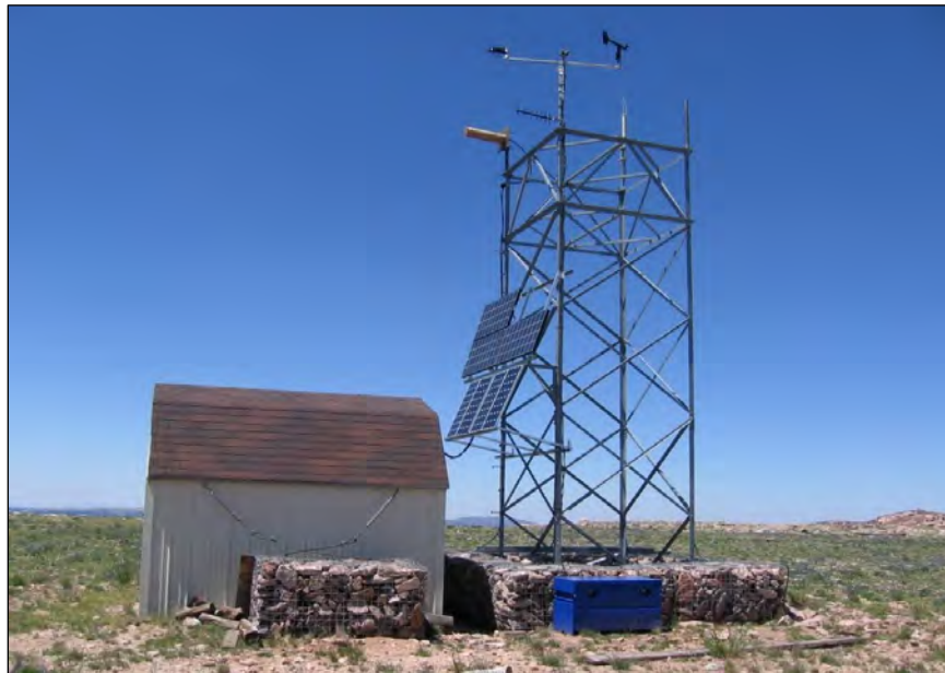
Figure 2.4 Icing Rate Meter Installation at the Dry Ridge Site
