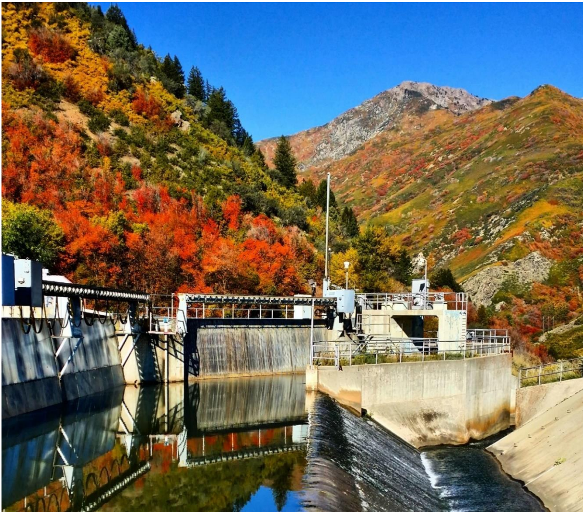
Diversion structure in Weber Basin
