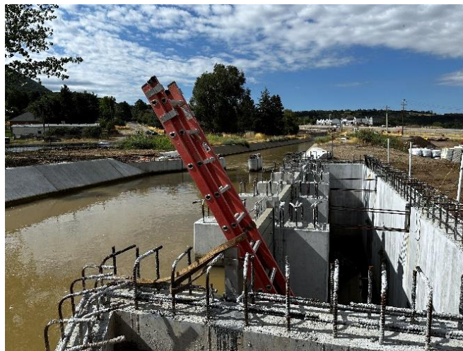
Aqueduct construction work in Weber Basin
