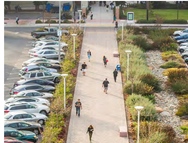
Parking lot adjacent bioswales reduce stormwater runoff and pollution (California State University, Fullerton, 2015).
