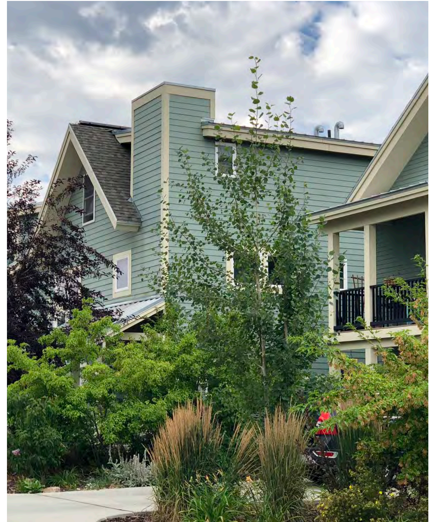
Snow Creek Cottages Affordable Housing
