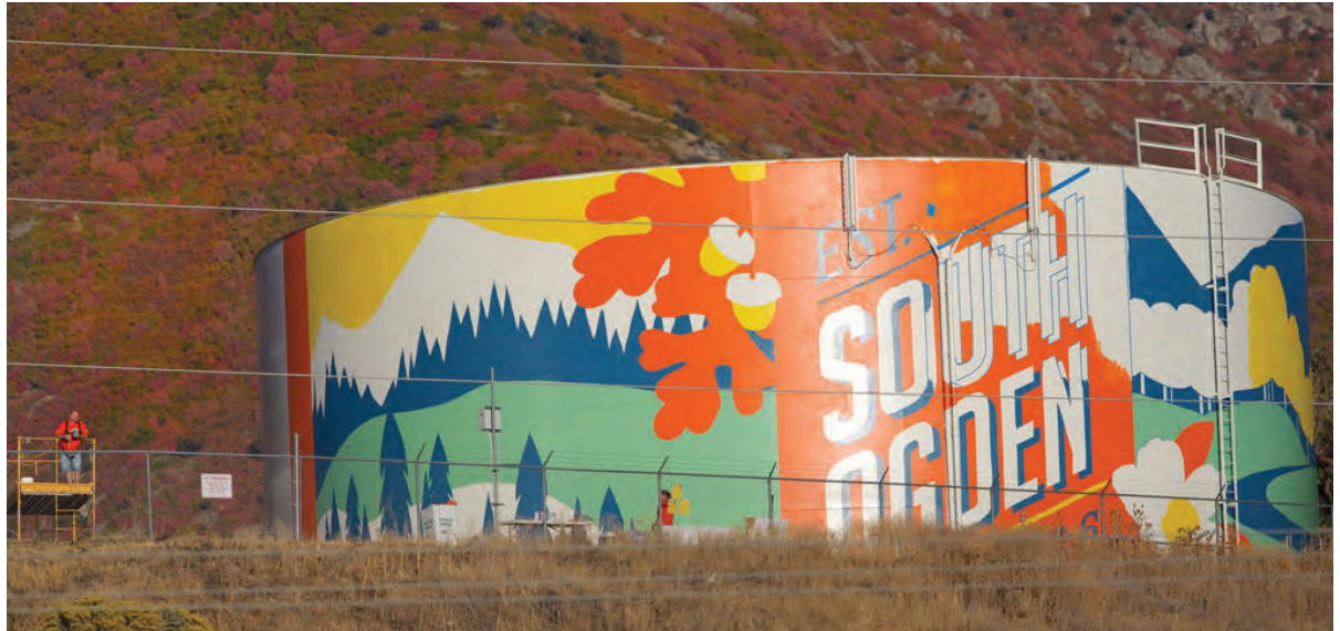
Caption: The South Ogden water tanks being painted as viewed from Harrison Boulevard on Wednesday, October 10, 2012. Credit: Dennis Montgomery/Special to the Standard-Examiner.
