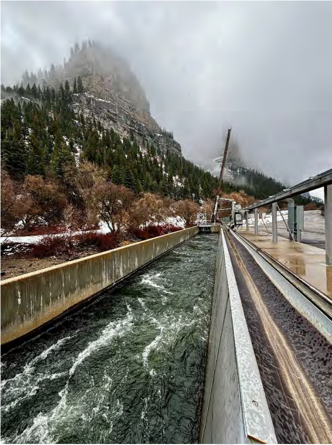
Olmstead Diversion. Photo credit Stephen Van De Graff.
