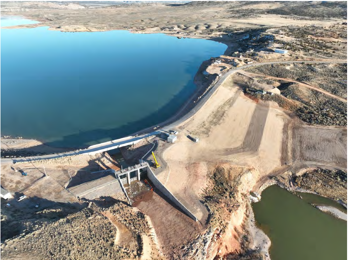
Rehabilitated Sevier Bridge Dam.
