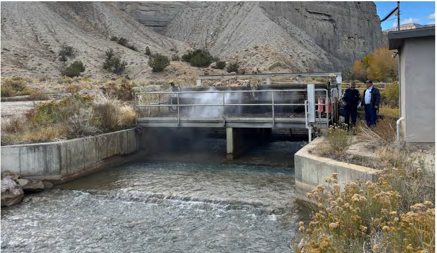
Automated and metered diversion. Photo credit Emery County Water Conservancy District.
